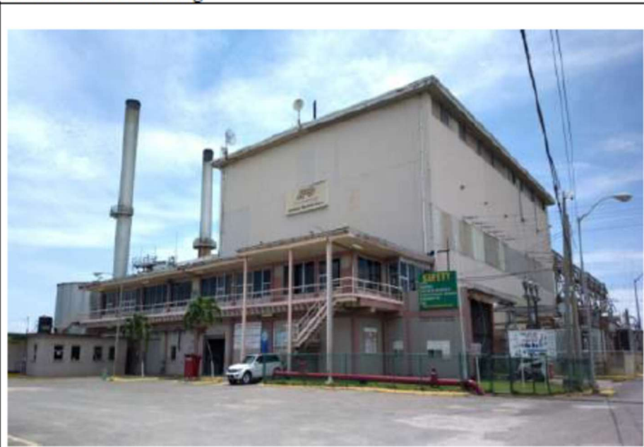
Photo 1 – Old Harbour Plant front and Admin. Building
