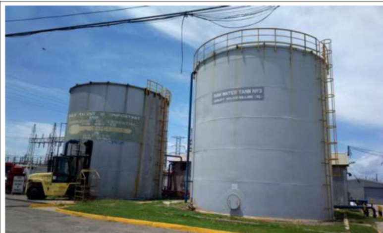
Photo 9 - Raw water tanks #1 and 3
