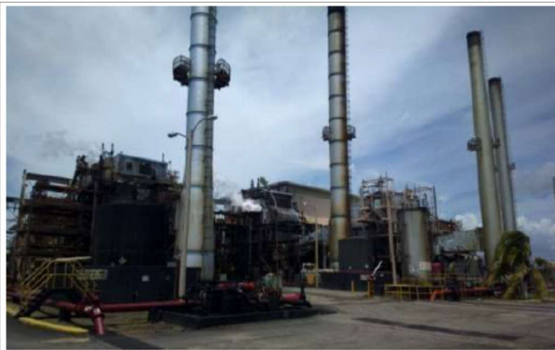
Photo 4 - Southern End of Plant Stack
