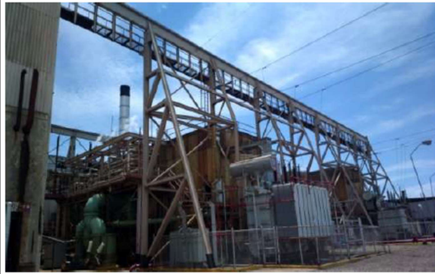
Photo 5 - Northern end of plant/crane structure
