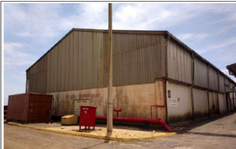
Photo 2 – Main Stores Building ( Concrete and metal sheeting)
