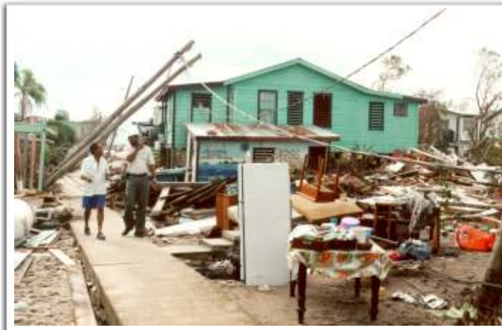
Above: Hurricane Iris ravaged Placencia Village causing significant structural damage and left many families homeless.
